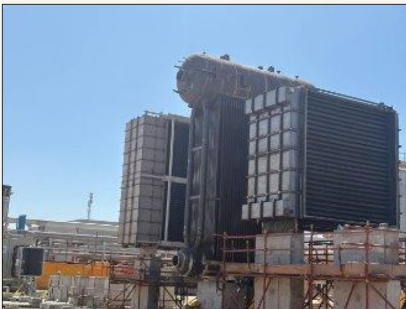
New CHP Plant during construction
